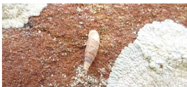
figure 4: ... and on the surface of the wall.
