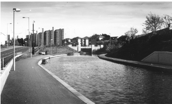
Fig. 2 The newly reconstructed stretch of the Union Canal at Wester Hailes, Edinburgh, showing the bare concrete banks and only very small patches of vegetation.
