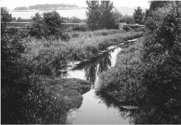
Fig. 4 The upper remaining section of the Monkland Canal near Calderbank, Lanarkshire.
