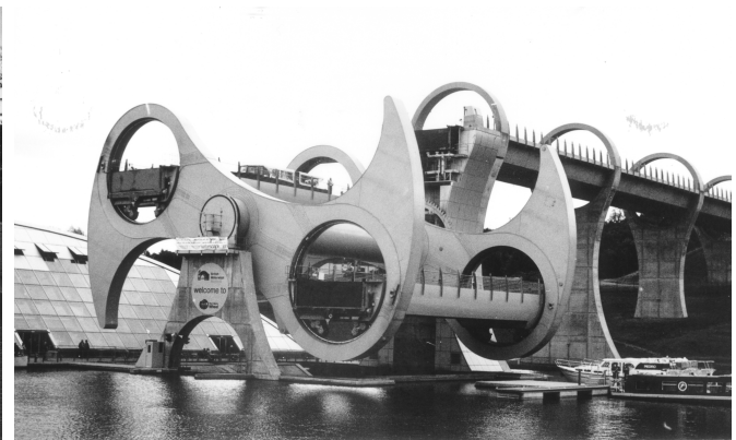
Fig. 3 The Falkirk Wheel. This structure, opened in 2002, is used to transfer boats, floating in sealed gondolas, from the upper level of the Union Canal to the lower level of the Forth & Clyde Canal. The Wheel is seen here in an intermediate position.
