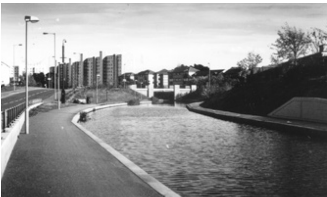
Fig. 2 The newly reconstructed stretch of the Union Canal at Wester Hailes, Edinburgh, showing the bare concrete banks and only very small patches of vegetation.
