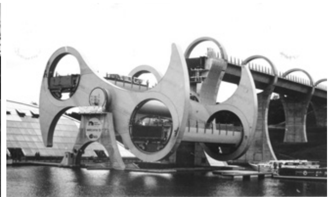
Fig. 3 The Falkirk Wheel. This structure, opened in 2002, is used to transfer boats, floating in sealed gondolas, from the upper level of the Union Canal to the lower level of the Forth & Clyde Canal. The Wheel is seen here in an intermediate position.
